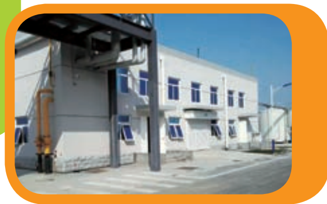
鍋爐房 Boiler Room
